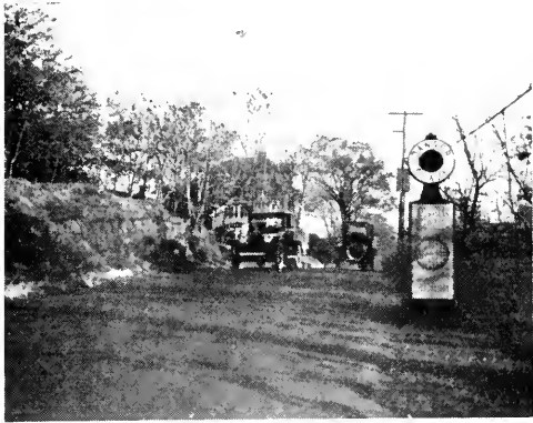
Typical flashing lighthouse on Maryland roads in the Twenties. It flashed the danger signal at the top of a hill. This one advertised golf balls.
